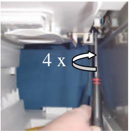
Screw the mechanism back on its place.
