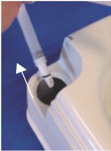
Bend the new flush tube into a horseshoe shape and place an elastic band around it half way down, forcing it to remain in this position.
