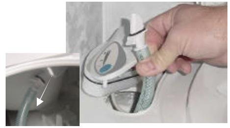
Disconnect the nozzle by pulling it (inside the toilet) down.
