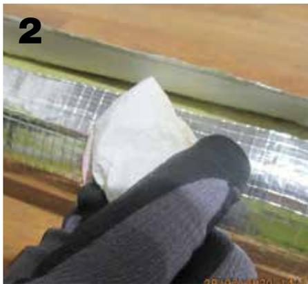
Before sealing, the mineral wool pipe section must be pressed together exactly. It is important to ensure that all adhesive points are free of dust, grease, and moisture before closing the adhesive tape!
