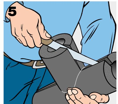
Using the K-FLEX® cutting board, cut the end of the shorter tube twice at an angle of 45°.
