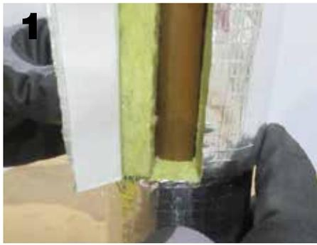
The mineral wool insulation pipe section with aluminum covering is slit on one side and can be wrapped around the pipe to be insulated.
