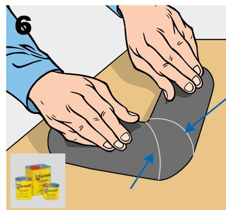
Cut the segmented elbow section along its length on the inside surface only.
